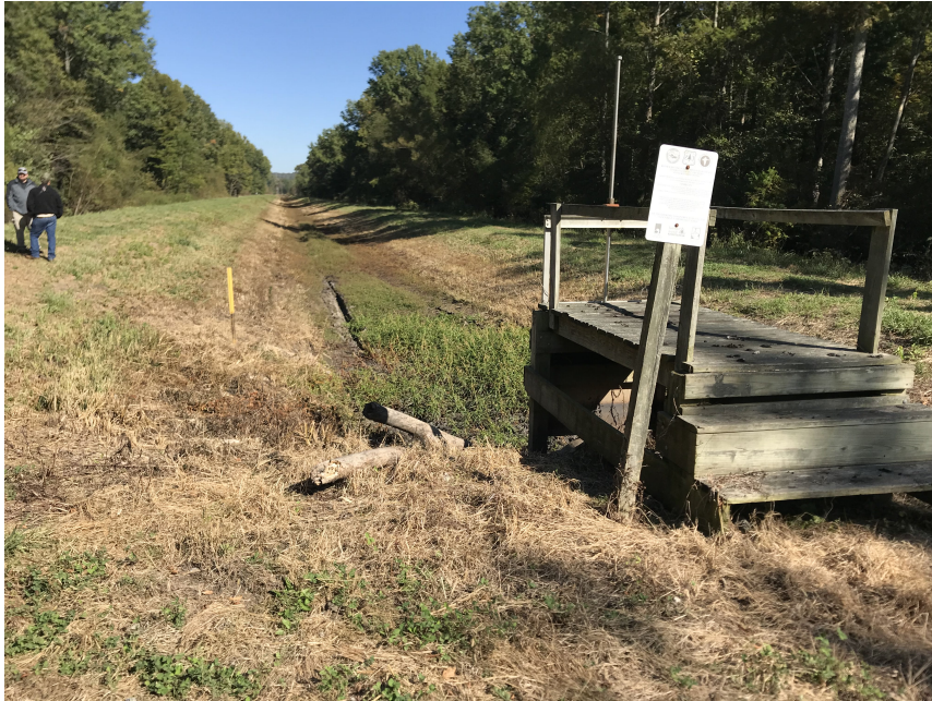
Figure 4 – Existing Berms with Channel in Center
